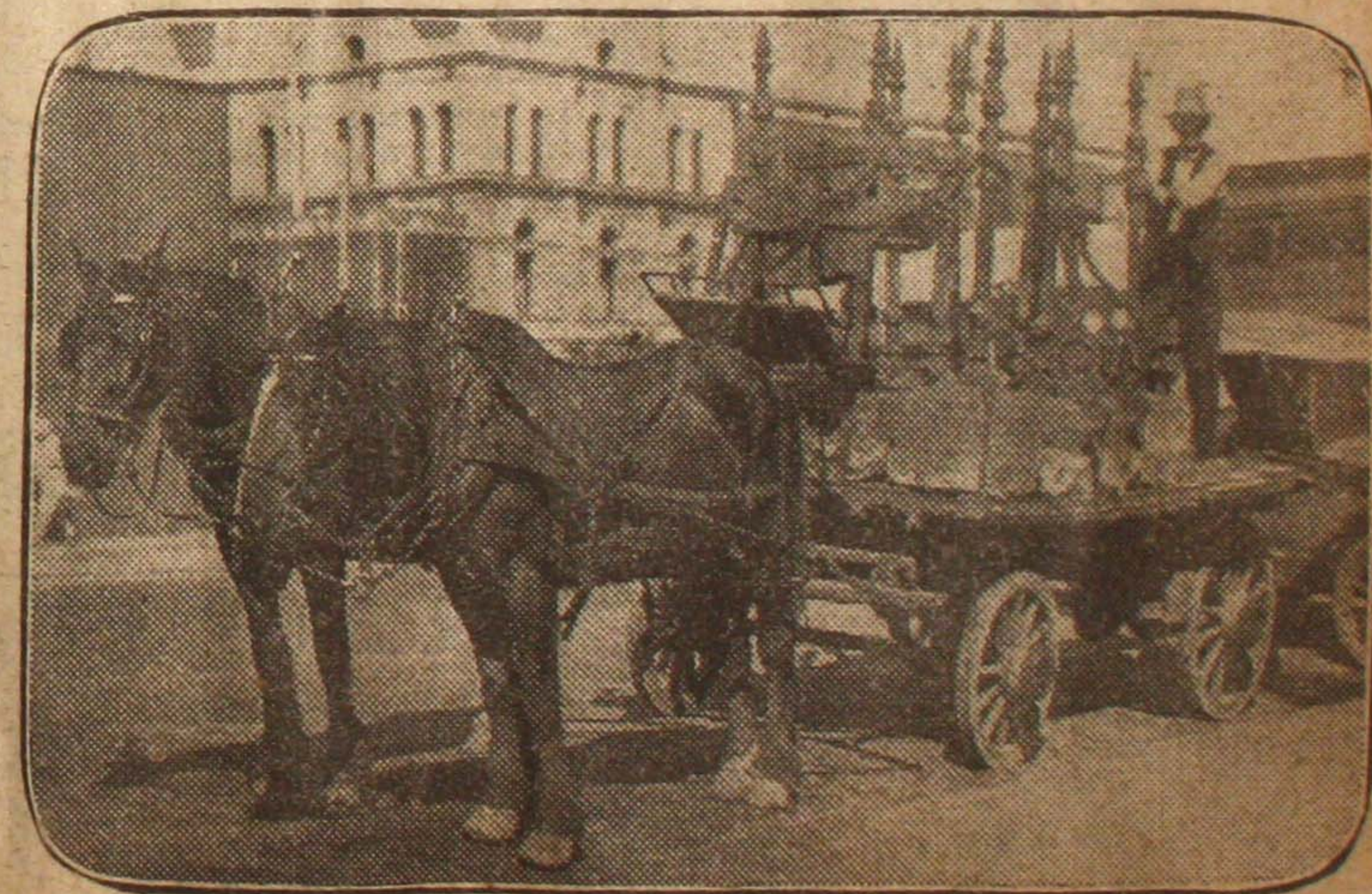
REMOVING THE VICTORIA SQUARE RAILINGS—A HOT JOB FOR A WARM DAY: To preserve the fence intact, the solder in the joints has to be melted out with the aid of firepots. This process is shown on the left. Right—Fence posts and their concrete foundations loaded on a lorry for transport to the University. In a few days this old-fashioned feature of the Square will have been entirely removed.
