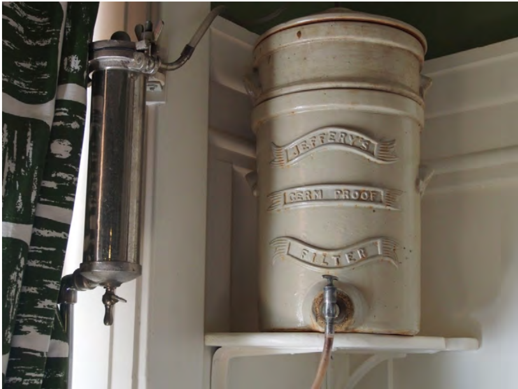
Figure 11. Jeffery's Germ Proof Filter in the working kitchen at Beleura Source: Photograph by Iain Buckland
