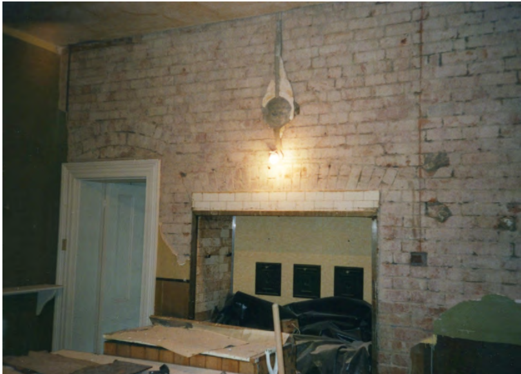
Figure 9. Alcove in French kitchen for cast iron stove – under restoration post-1996 Source: Beleura House & Garden Collection
