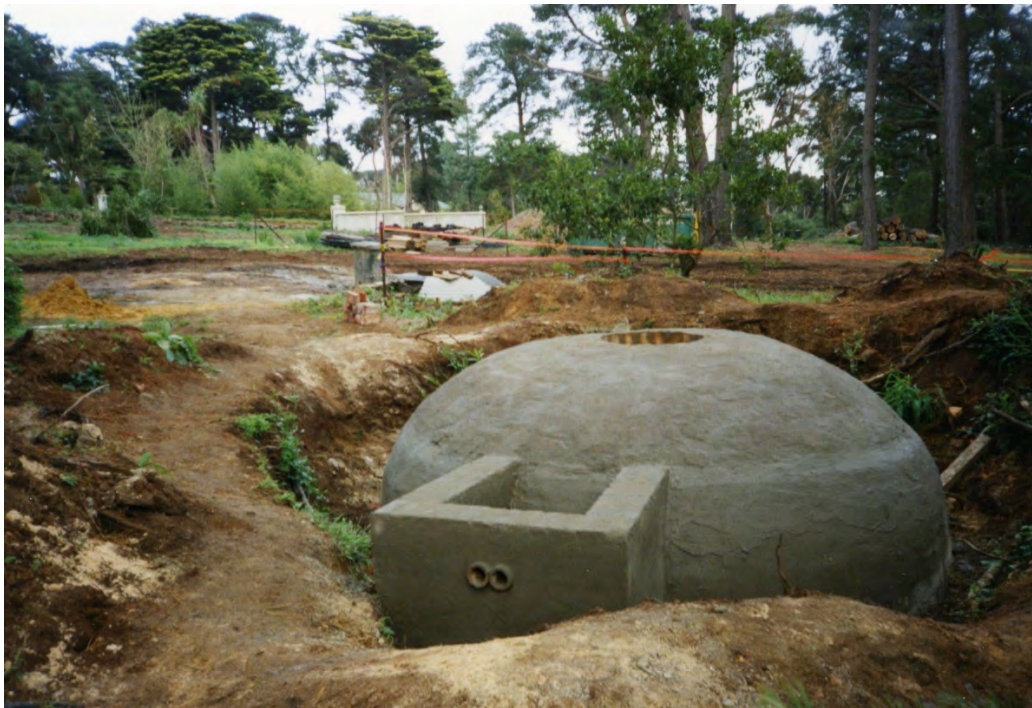
Figure 12. Underground brick water storage vessels with bell-shaped tops (under restoration) Source: Beleura House & Garden Collection
