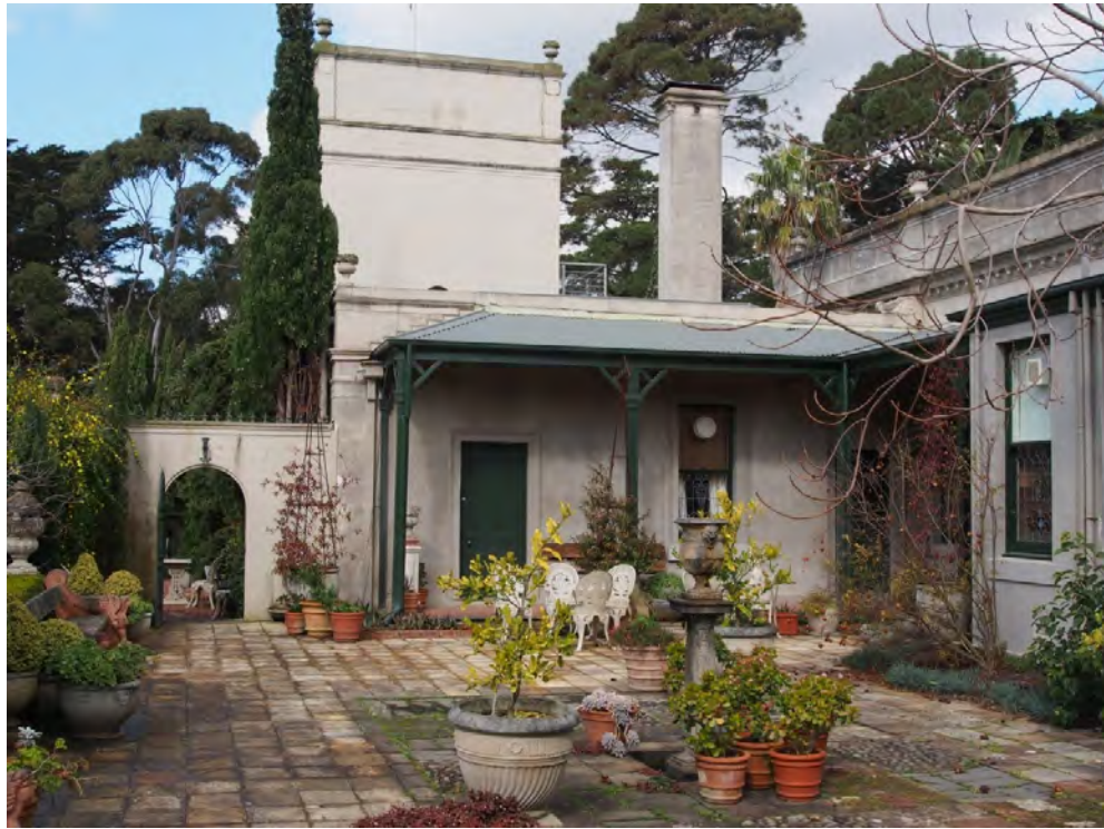
Figure 13. Beleura tower and enclosed water tank above eastern courtyard Source: Photograph by Iain Buckland
