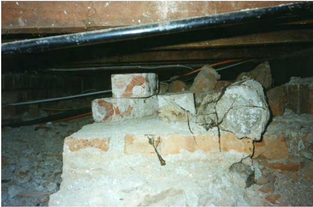
Figure 8. Remnants of brick piers from early detached building under floor of current French kitchen Source: Beleura House & Garden Collection
