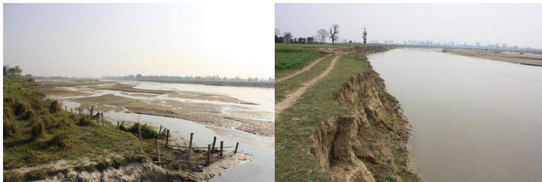
Plate 6.4 Bamboo piling to protect land from floods in Damak (left). River water eroding agricultural fields in Dhangadhi (right).
