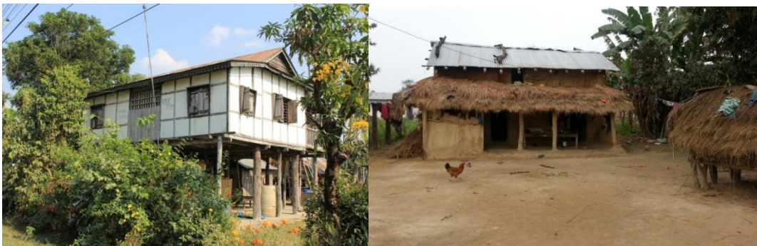
Plate 4.4 Left: A typical wooden post house in Damak. Right: A typical mud-plaster walled house in Dhangadhi.
