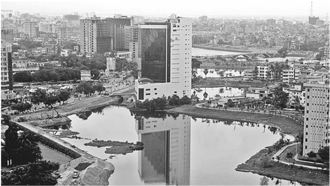
Figure 7-5: BGMEA building in 2016 (source: The Daily Star, http://www.thedailystar.net/city/sc-upholds-bgmea-building-demolition-order-1233319 )
