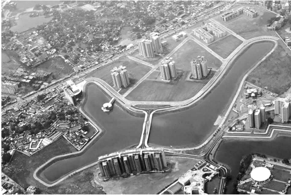
Figure 8-17: The Dhamalkot military residential development (source: Bangladesh Airforce)
