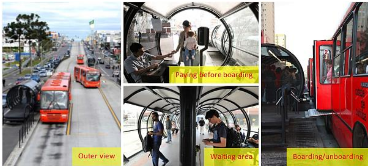
Figure 7.10: Typical Curitiba tube station (Source: adapted from Lindau et al. 2010; Reed 2015)
