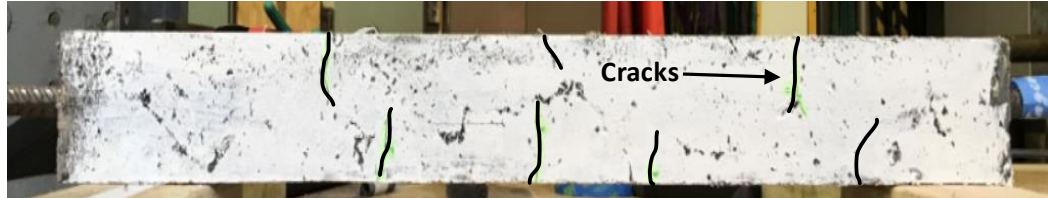
Fig. 4.7 The formation of cracks from tension stiffening test at 28 th day.
