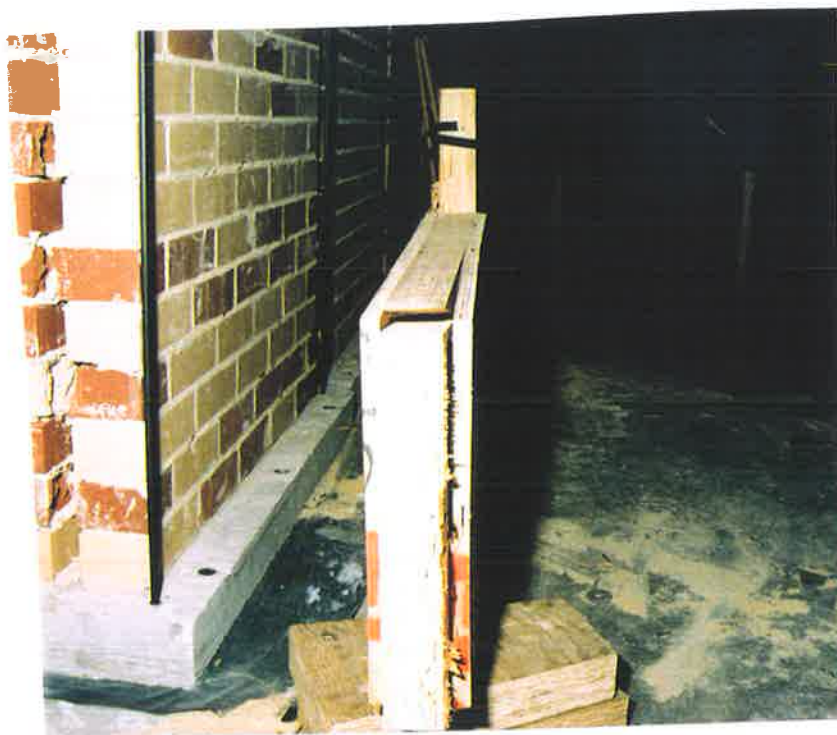
Figure 5.48 Failure mode of specimen 7
