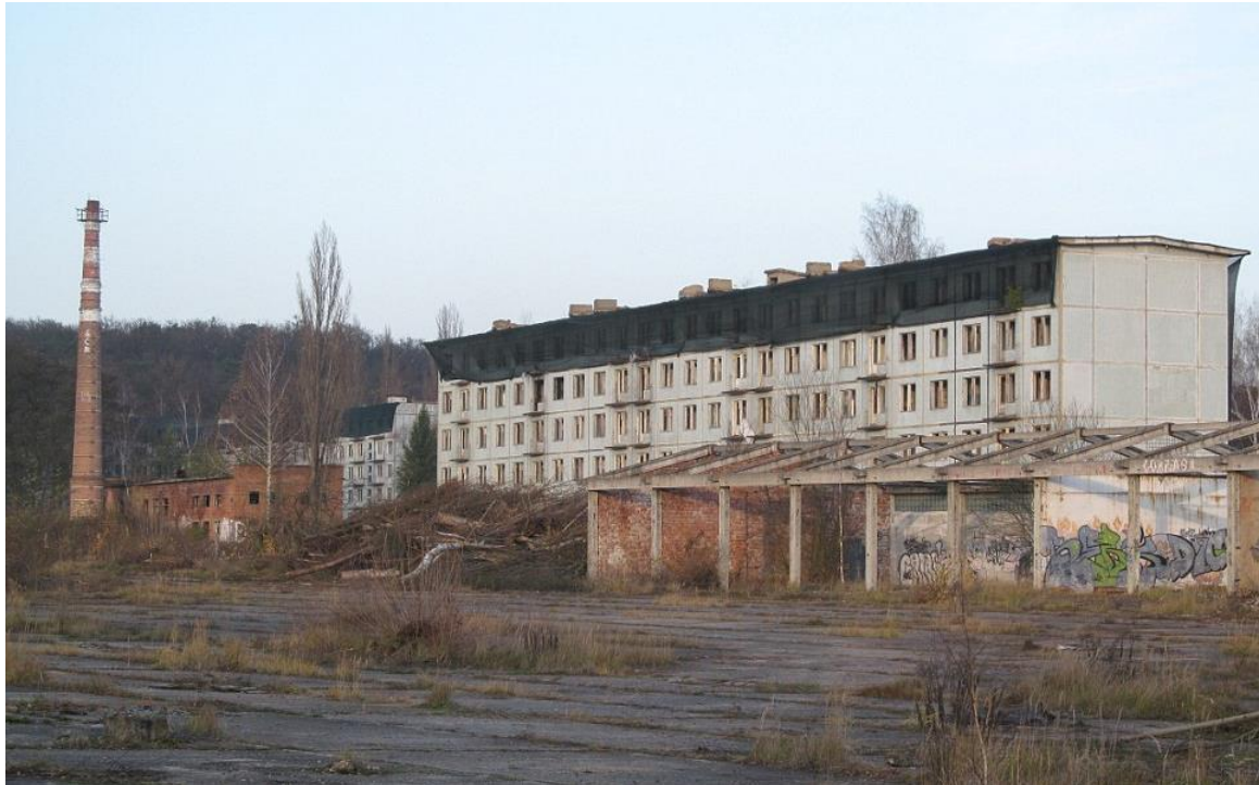
Figure 5.4 An abandoned and evacuated military brownfield site in Boží Dar, former Czechoslovakia (Source: http://www.dailymail.co.uk/ ).
