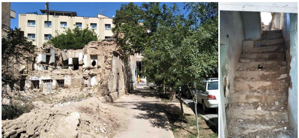
Figure 10.6 Former residential site having been left dilapidated and abandoned for many years in an inner-urban area in Shiraz ( Photos were taken by the author in May, 2018 ).
