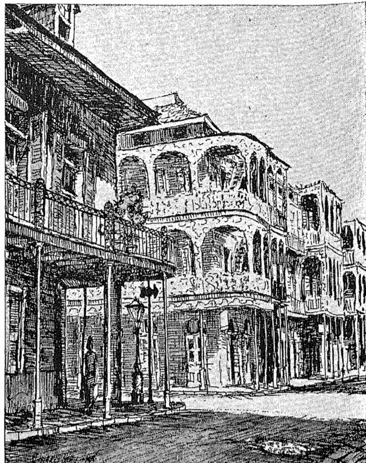
Cast Iron of the French Quarter—St. Peter's Street, off Bourbon Street.
