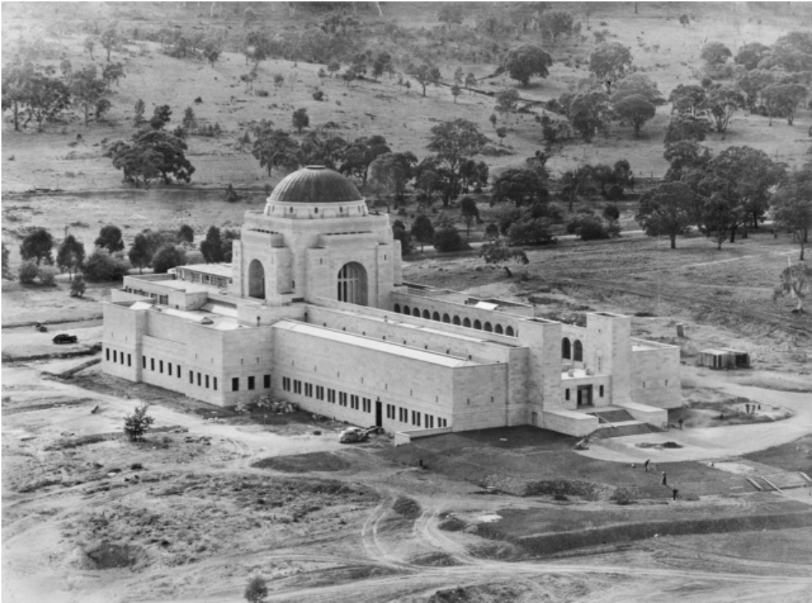
Fig. 3.2. Aerial view of the Australian War Memorial from the north-west (c.1940-1941). 54
