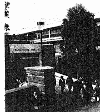
The Barr-Smith falls short on disabled access.
