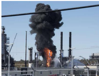
Figure 1.1 Release of flammable gas due to the damage of a butane oil pipeline [6]
