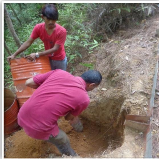
Plate 7: Groundworks for overland flow system at the PF site
