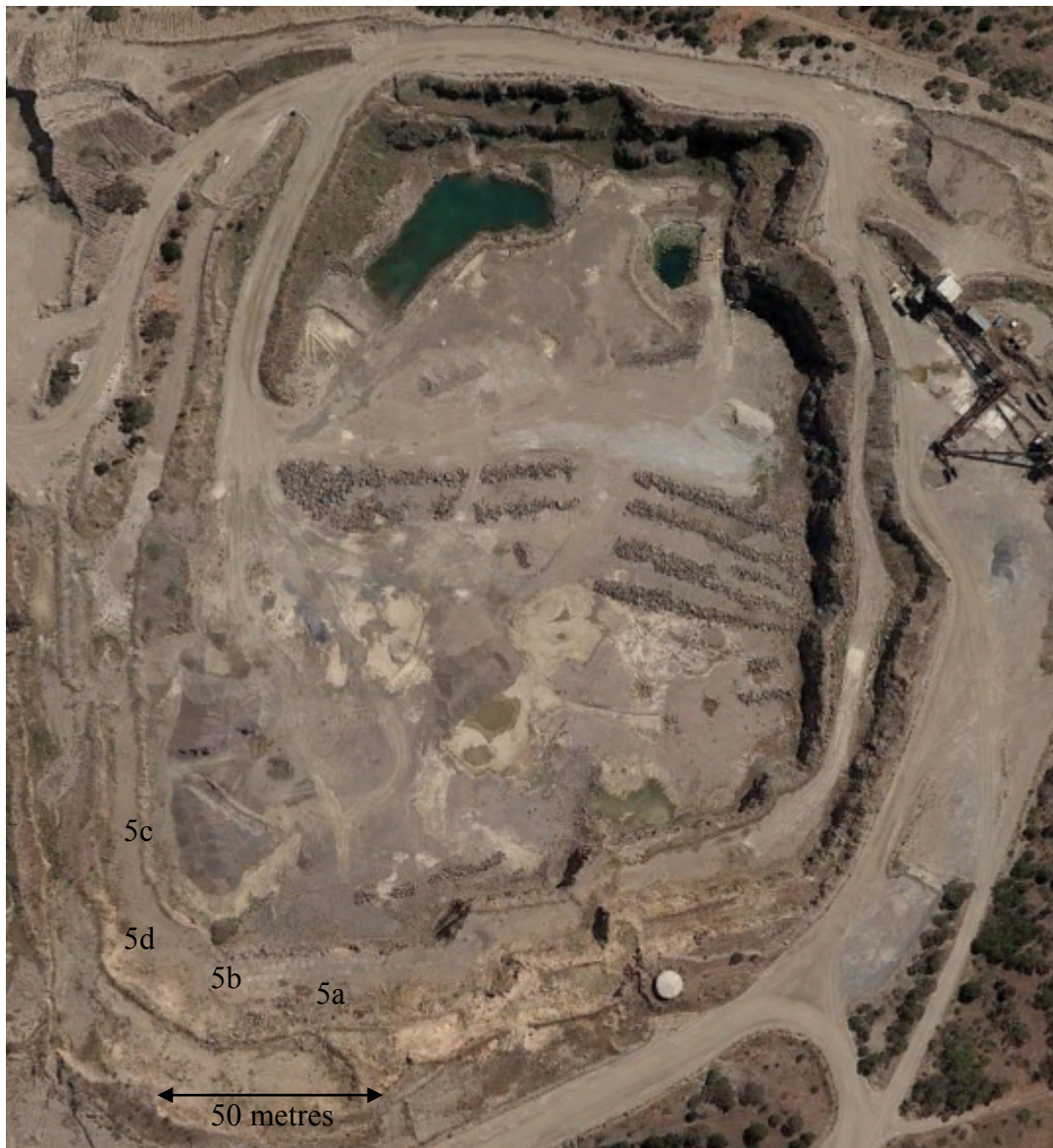
Image 5e: Birdseye view of Murray Bridge Quarry displaying the mapped quarry faces
