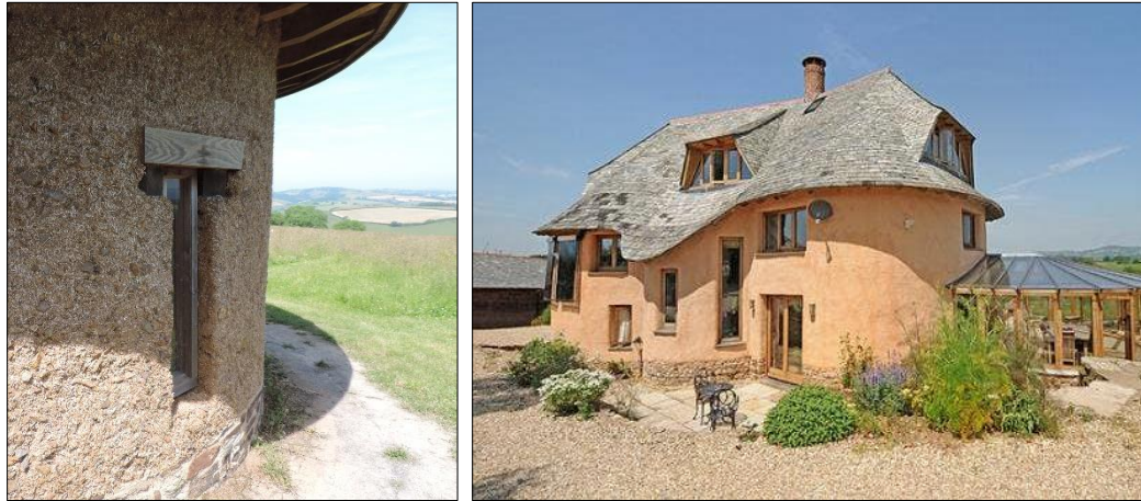
Figure 6. Cob building in Totnes, UK (Veliz Reyes et al. 2018) (left); and Keppel Gate cob house in Devon, UK by Kevin McCabe (McCabe 2020)
