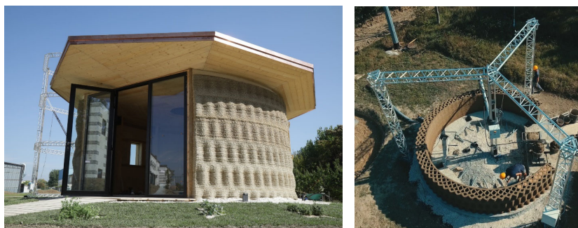
Figure 2: 3DP cob house fabricated by WASP3D.
