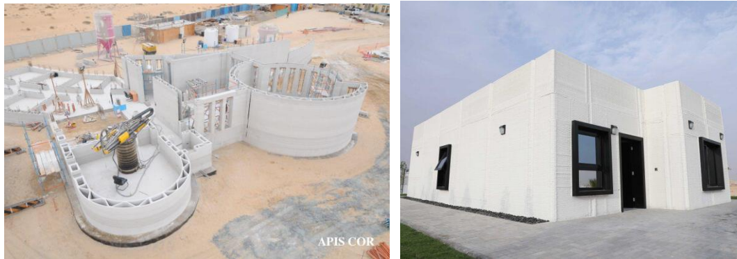
Figure 4. 3DP building in Dubai by Apis-cor (Apis-cor 2019)(Left) and 3DP house in Saudi Arabia by CyBe (CyBe 2019) (Right).
