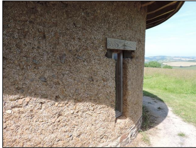
Figure 1. Exposed cob construction in Totnes, UK.
