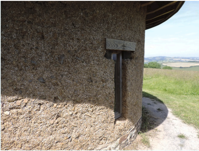
Fig. 1. Exposed cob construction in Totnes, UK.
