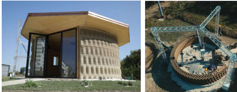
79 80 Figure 2. 3DP earth house by WASP 3D.
