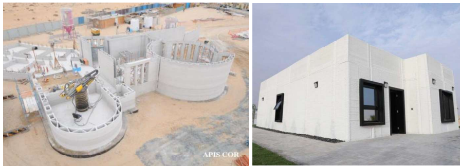
51 52 Figure 1. 3DP building in Dubai by Apis-cor (Left) and 3DP house in Saudi Arabia by CyBe 53 (Right).
