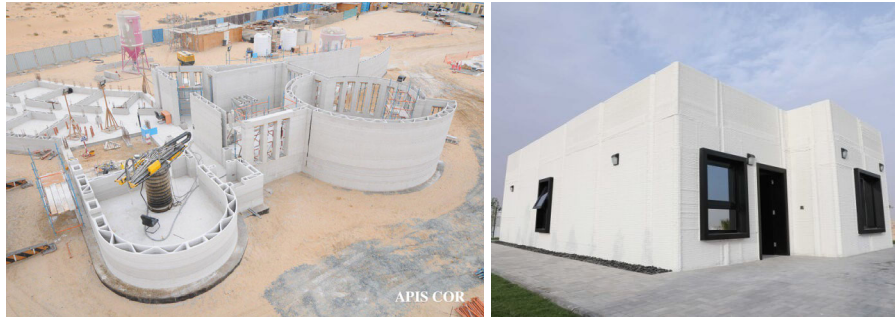
Figure 1: 3DP concrete building in Dubai by Apis-Cor (Left) and 3DP house in Saudi Arabia by CyBe (Right).
