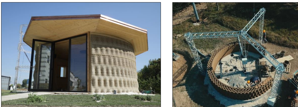
Figure 7. Earth house prototype by WASP in Italy (left), and the 3D printing system of earth (Right)(3D-WASP 2020).
