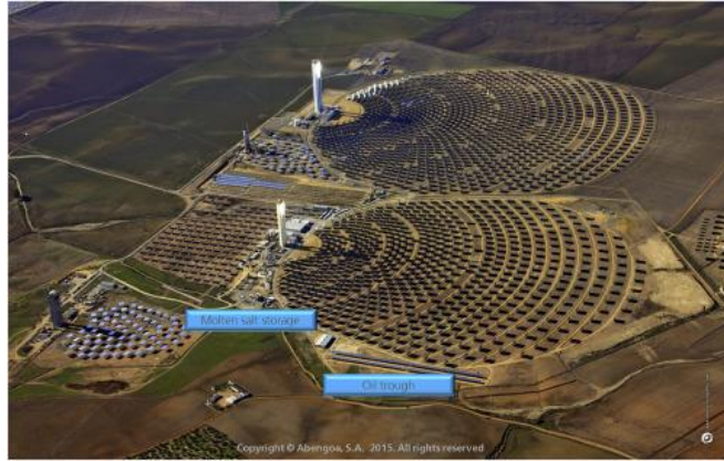
Figure 1.5- Aerial view of Solucar Solar Platform in Spain by Abengoa, featuring tower mounted solar cavity receivers and heliostat field (Prieto et al., 2016).
