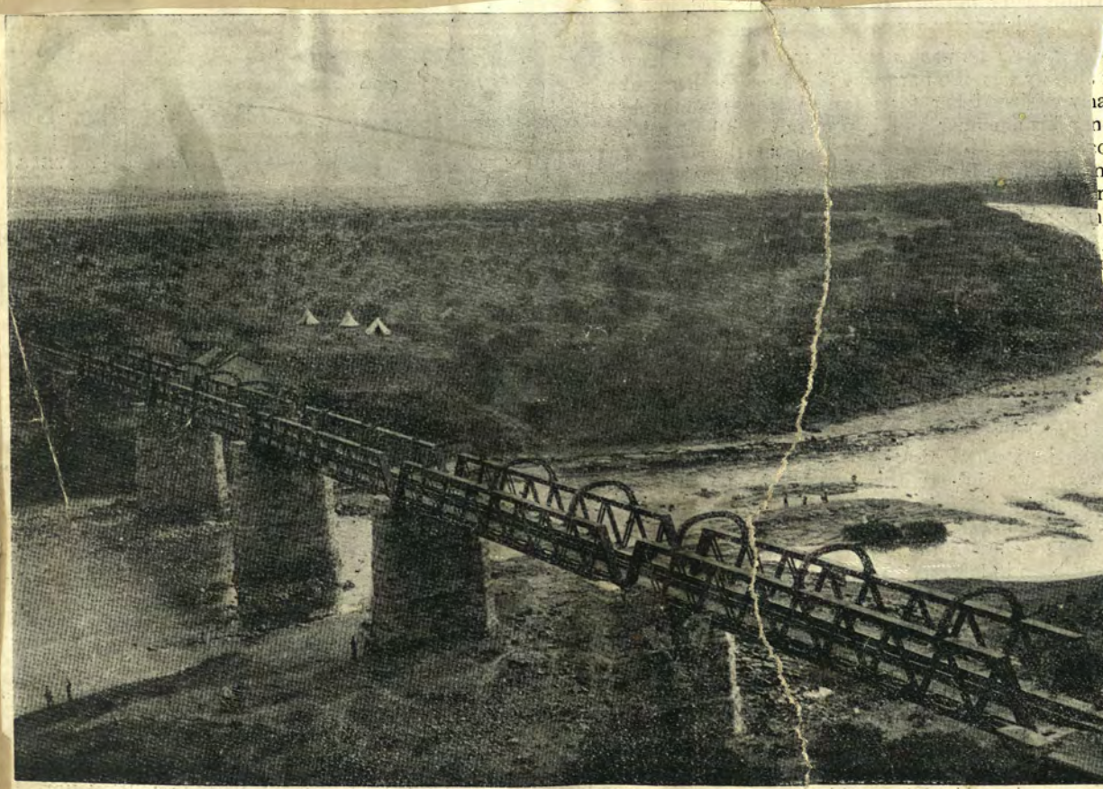
COLENZO BRIDGE ACROSS THE TUGELA.
