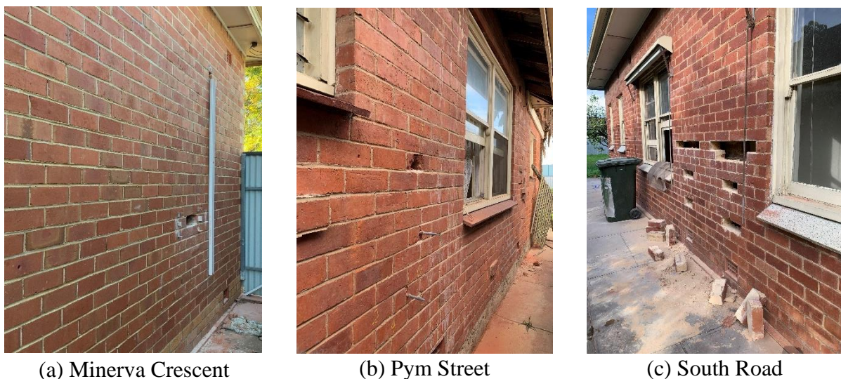
Figure 1 – Typical masonry at each site
