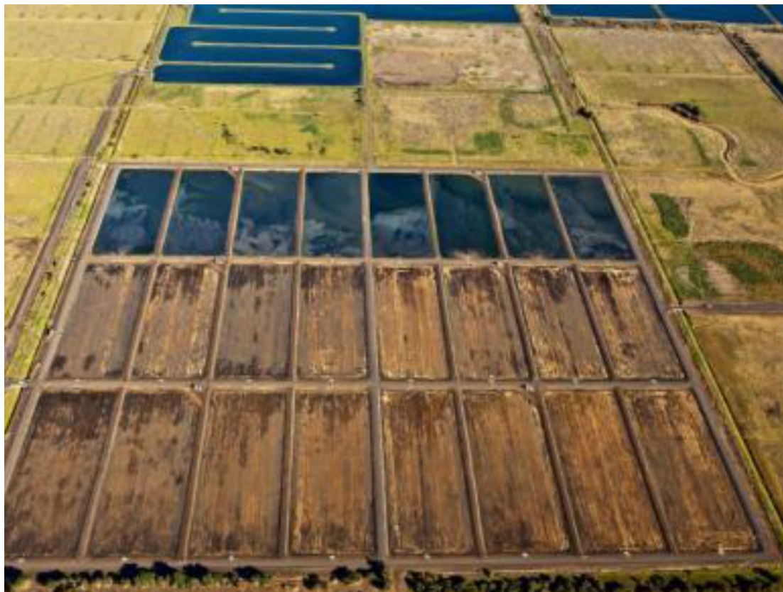
Figure 3: Biosolids stockpiles at the Western Treatment Plant in Werribee, Victoria Australia 168 .
