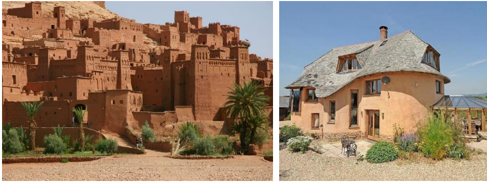
Figure 2. Examples of traditional earth-construction. Adobe houses of the Kasbah at Ait Benhadou in Marrakesh, Morocco (left)(Ahmed and Ibrahim, 2018), and Keppel Gate cob house in Devon, UK (right) (McCabe, 2020).
