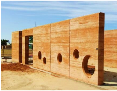
Figure 4. Kalkee Road Children's & Community Hub by Rammed Earth Enterprises® (2019).
