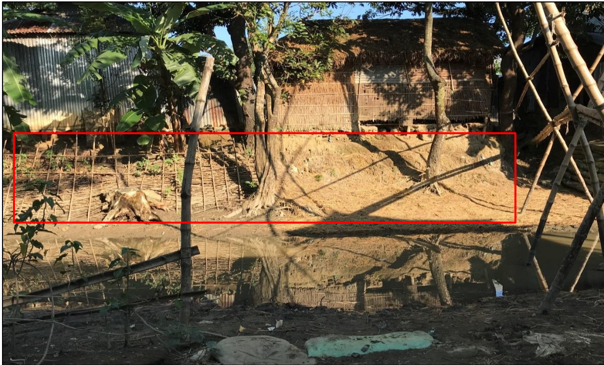
Plate 7.1 Use of rice straw to prevent the erosion of settlement area in flood-hit village (Lamagaon).
