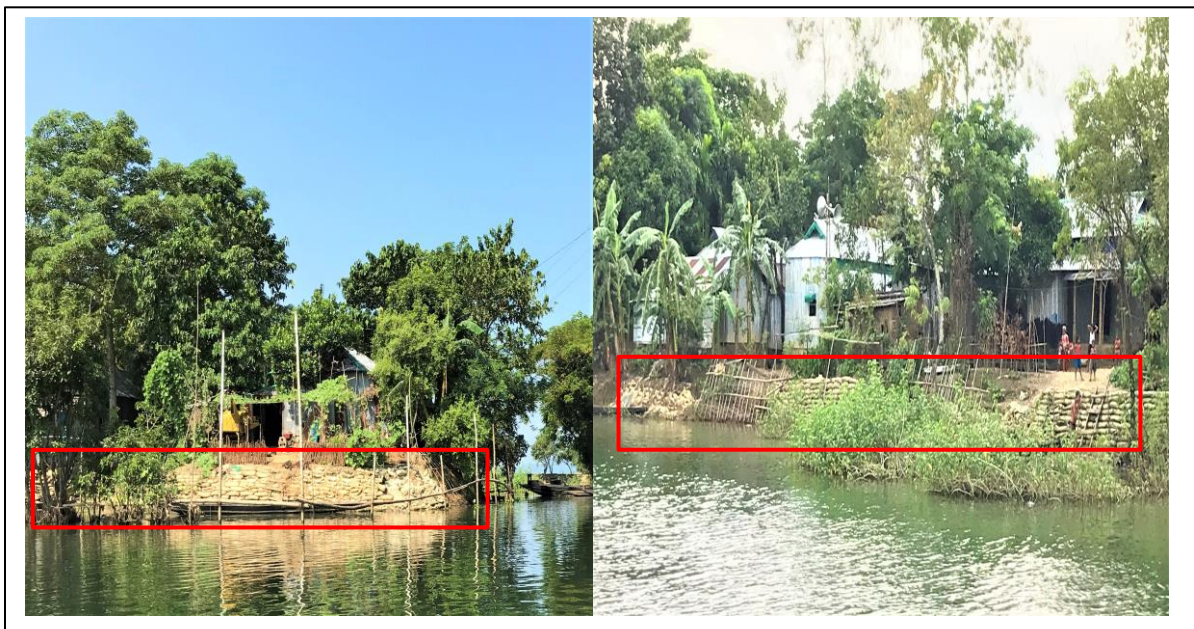
Plate 4.1 Temporary protective walls around the settlement in flood-affected village of Lamagaon.
