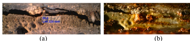
Fig. 9. (a) Crack before immersion, (b) healing of crack after 24 weeks immersion.
