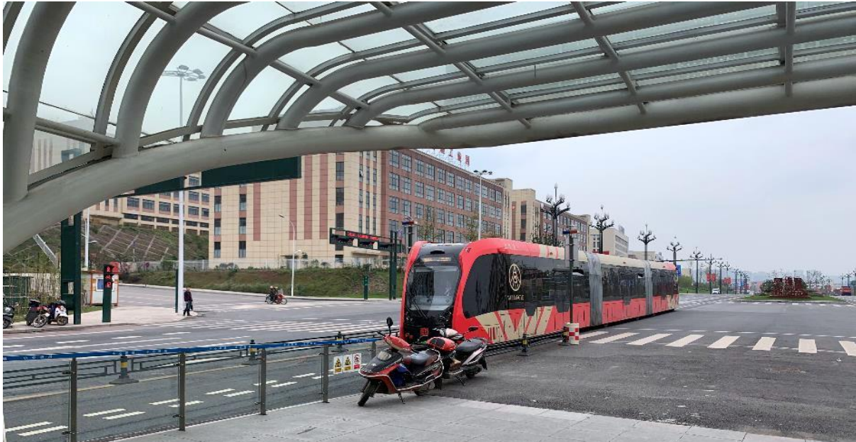
Figure A2-3: ART arriving at ART Industry Park Station along wide, multi-lane main road located in the outer urban area (Source: Daniel Conley)
