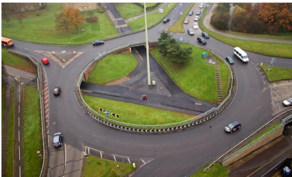
Figure 8-2: An example of Stevenage’s grade-separated cycling infrastructure that avoids interaction with traffic (Source: Carlton Reid, The Guardian)
