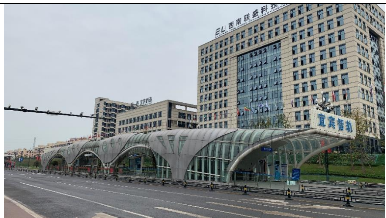
Tram/BRT like station at ART Industry Park Station
