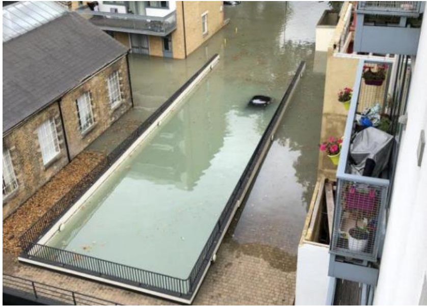
Figure 5-18. A large car park was flooded due to the pipe burst.
