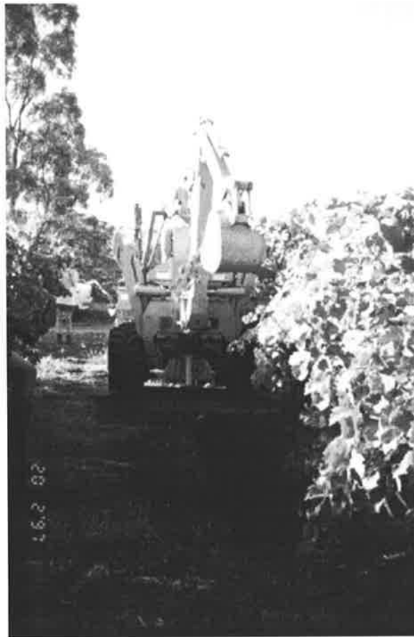
Figure 7.7 Backhoe at work between the vines at the Overland Corner site
