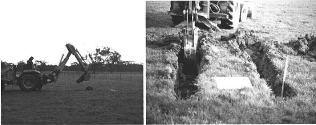
Figure 7.1 The back-hoe at work at the Rutherglen site
