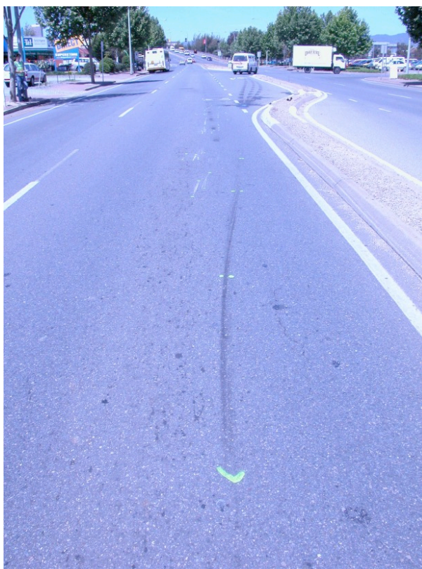
Figure 3.2 Crash site for M154 showing the right turn lane and tyre marks associated with the crash
