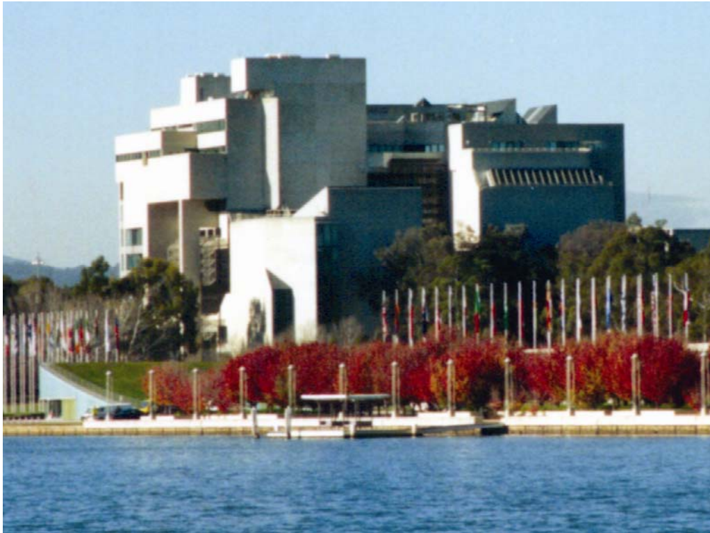
Figure 6 High Court Building, Canberra, ACT.
