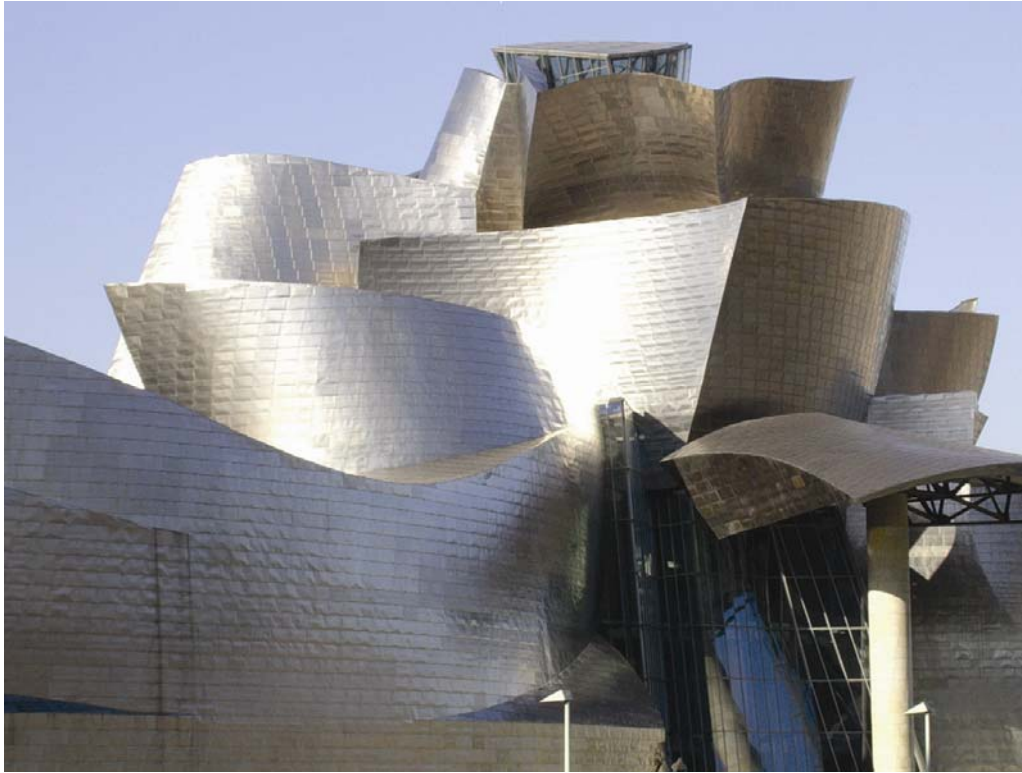
Figure 3 GMB, View from the bridge.
