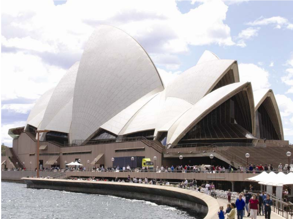
Figure 15 Sydney Opera House, Bennelong Point, Sydney.
