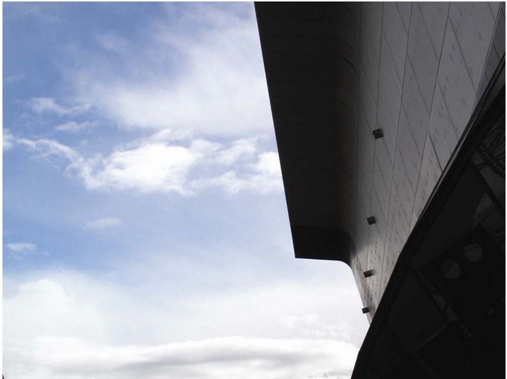
Figure 28 NMA, Parapet, Main Hall.
