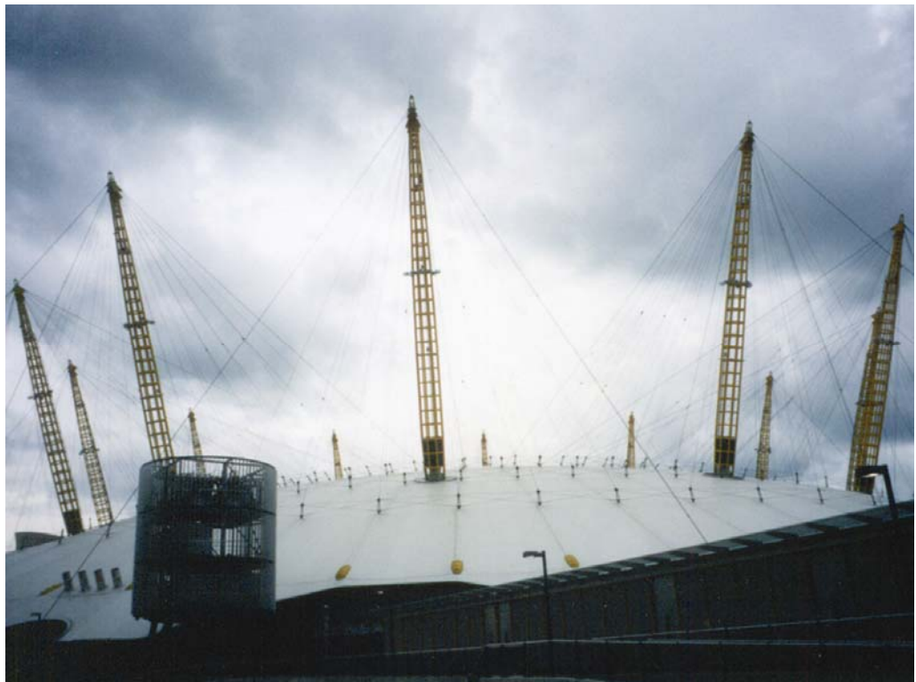
Figure 12 Millennium Dome, Greenwich, London.
