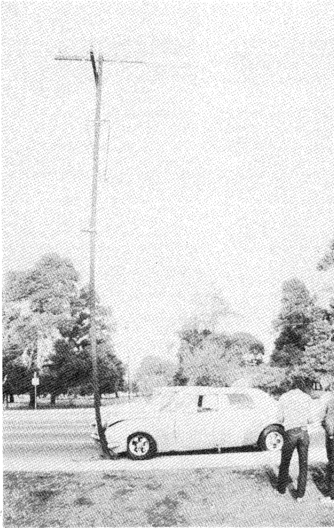
FIGURE 3.21: Damage to pole, Accident 100. (see Figure 3.20)
