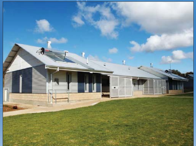
The Mobilong independent living units were designed using reverse veneer and solar power to reduce long-term operating costs.
