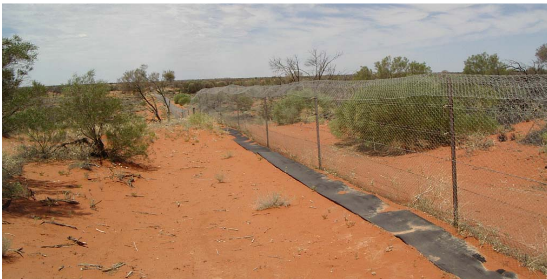
Figure 2.1: A view from outside showing the 1.8 m high predator-proof fence with floppy top, foot apron and two electric wires. The electric wires are only on the initial fence around the Main enclosure. Rubber matting and/or wider netting has been used on top of the 30 cm foot apron in areas of erosion-prone dunes and watercourses to prevent rabbit incursions (Moseby and Read 2006).
