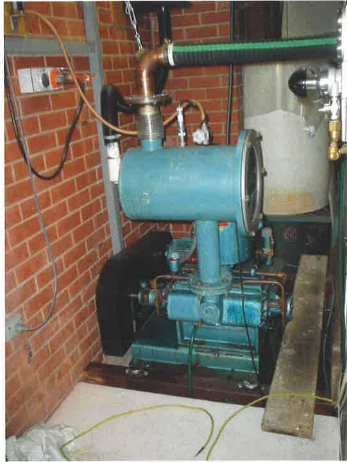
Figure C.3: Photograph of the roughing pump. Pumping is through the green striped black rubber pipe at the top of the picture. The pump exhaust is vented through the large black pipe on the left of the photo to a vapour trap and then expelled from the pump-room by an exhaust fan.
