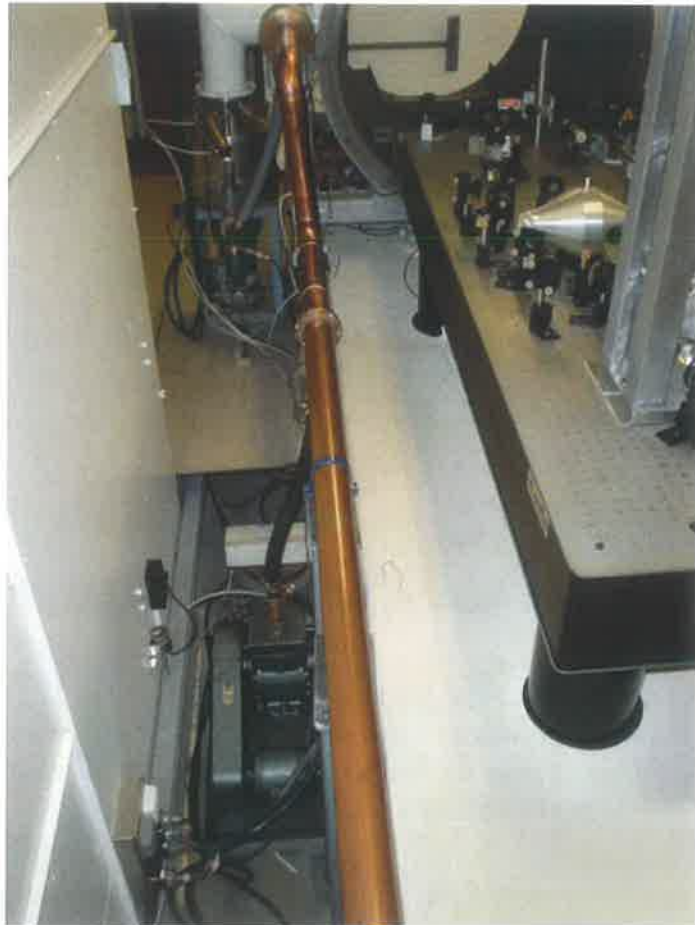
Figure C.4: Photo showing the small backing pump in the trench at the bottom-left of the picture.
