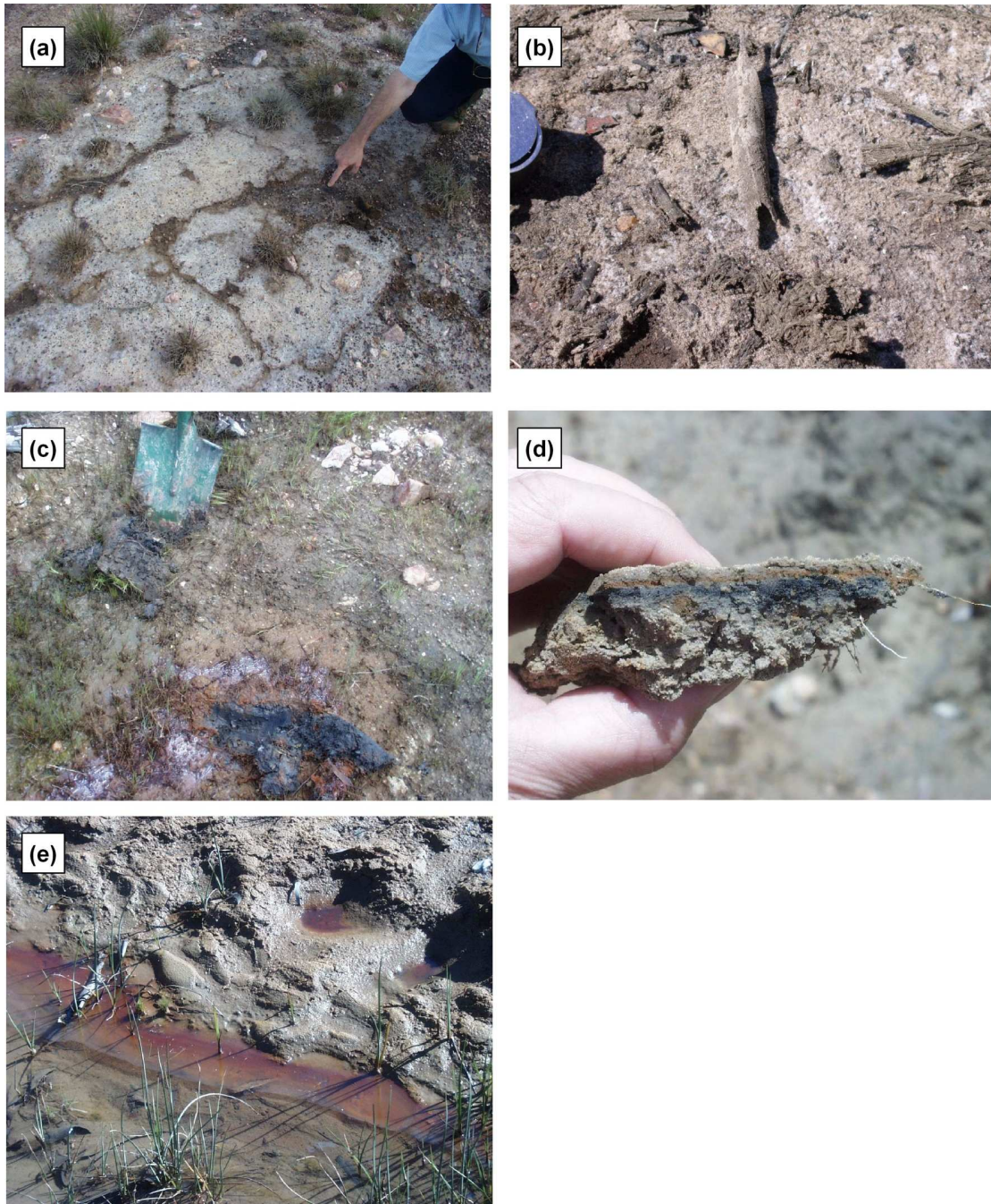
Figure 9.14. Plate (a) showing eroded surface fissures, which seep saline groundwater under piezometric pressure, in salt encrusted sodic surface clays in scalded lower landscape zones. Plate (b) shows surface salt crusting in highly saline (e.g. EC_{se} > 30 dS/m) topsoil. Plate (c) shows salt-iron crusts and exposed mono-sulfidic back ooze in the near-surface, and Plate (d) shows the layering in profile. Plate (e) shows the release of iron-rich gelatinous precipitates (featuring ferrihydrite) to Herrmanns Creek.
