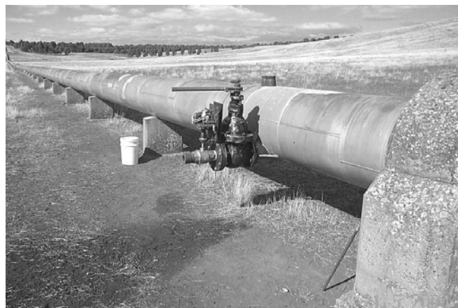
Figure 5-1 – Typical saddle supports for transmission pipeline (with collar restraint at right hand edge of picture)
