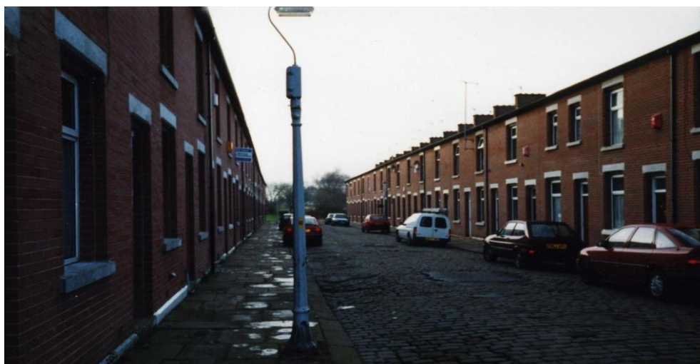
Figure 10. LJ's street after renovations, 2005.
