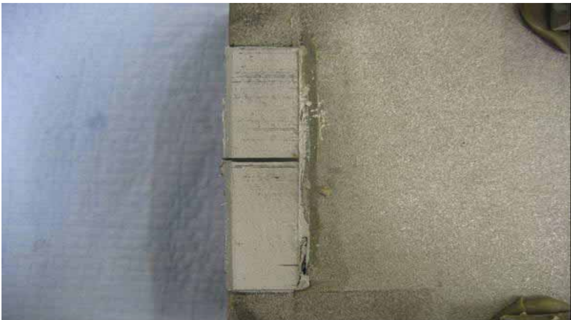
(b) Adhesive layer at failure
