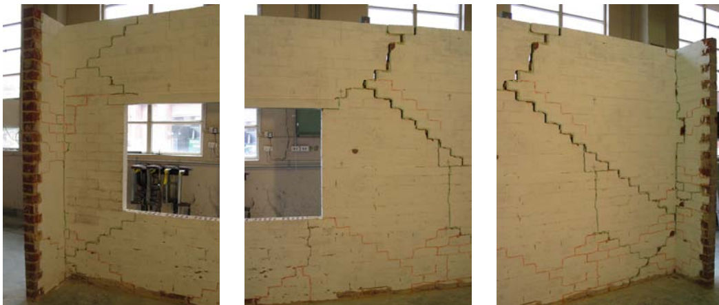
Figure B.37: Photograph of wall S6 crack pattern at the conclusion of cyclic testing.
