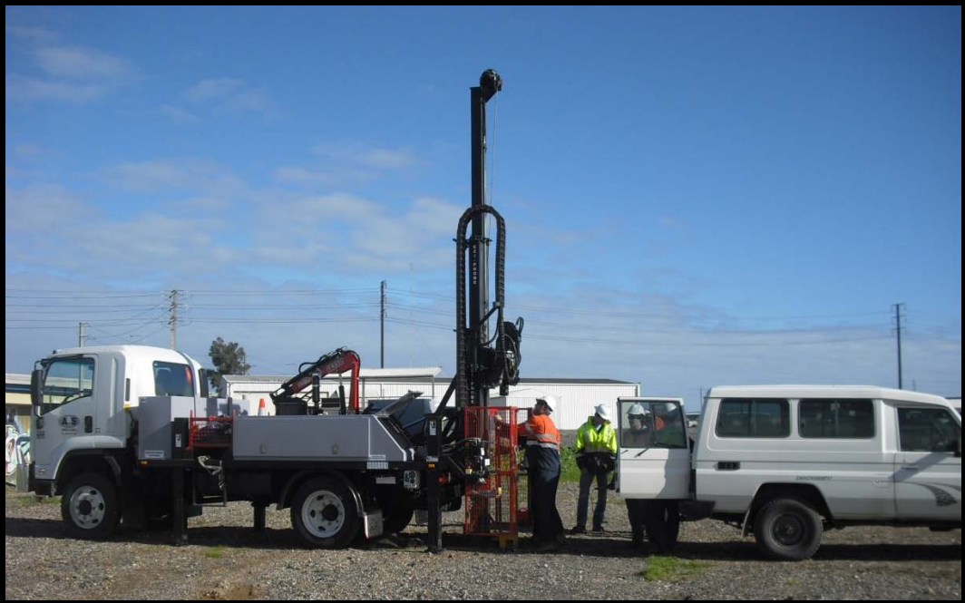
Figure 3.15 CPT in-situ testing activities at CPT #1
