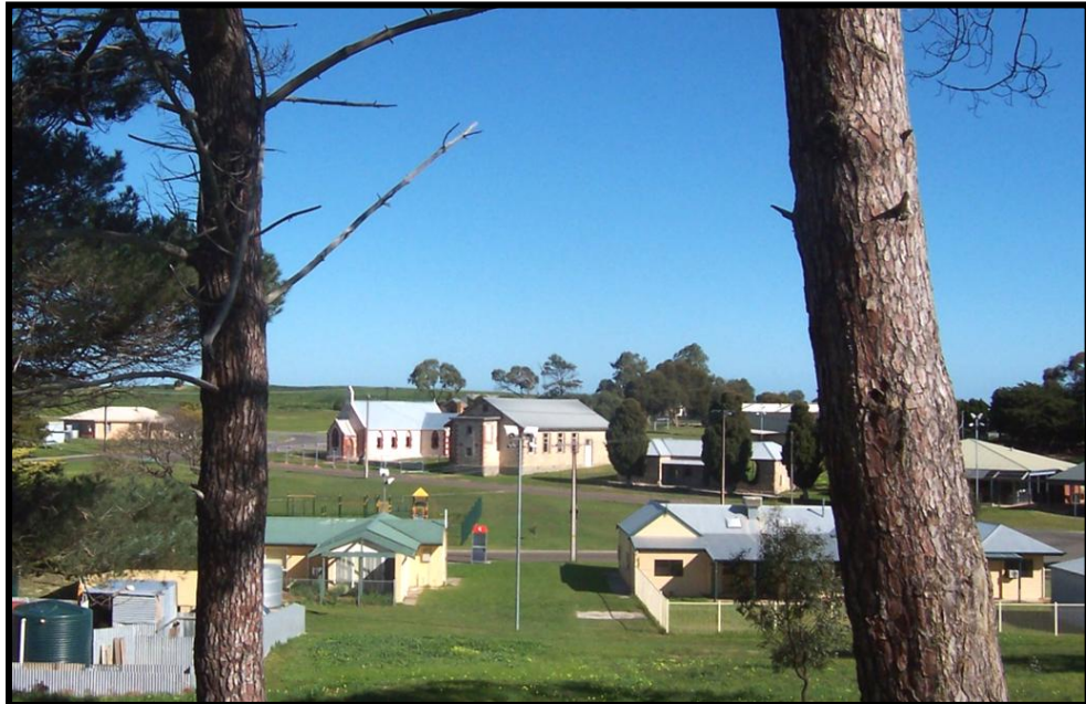
Figure 29: Raukkan looking towards chapel 2007. (C. Lockwood)
