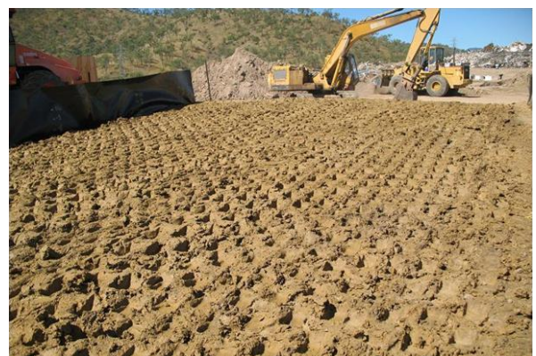
Figure 4.23 Phytocap Lysimeter (left) and Compacted Clay Barrier (right) During Construction (Photos courtesy of G. Zhu)
