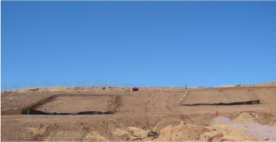
Figure 4.8 Completed Material Placement and Berm Construction of SWD Trial Site
