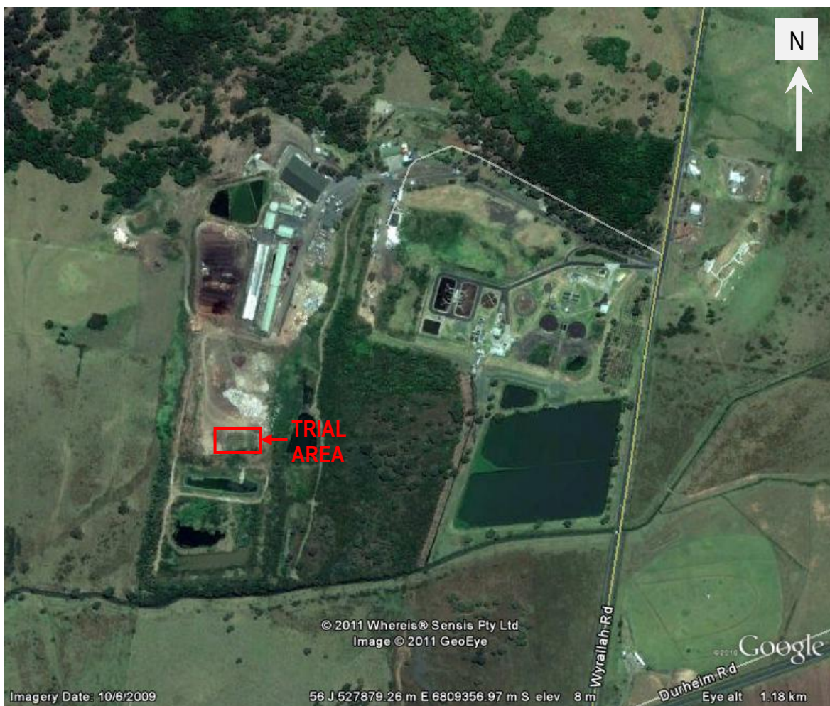
Figure 4.25 Lismore Waste Facility and Trial Area (Source of base plan: Google, 2011)
