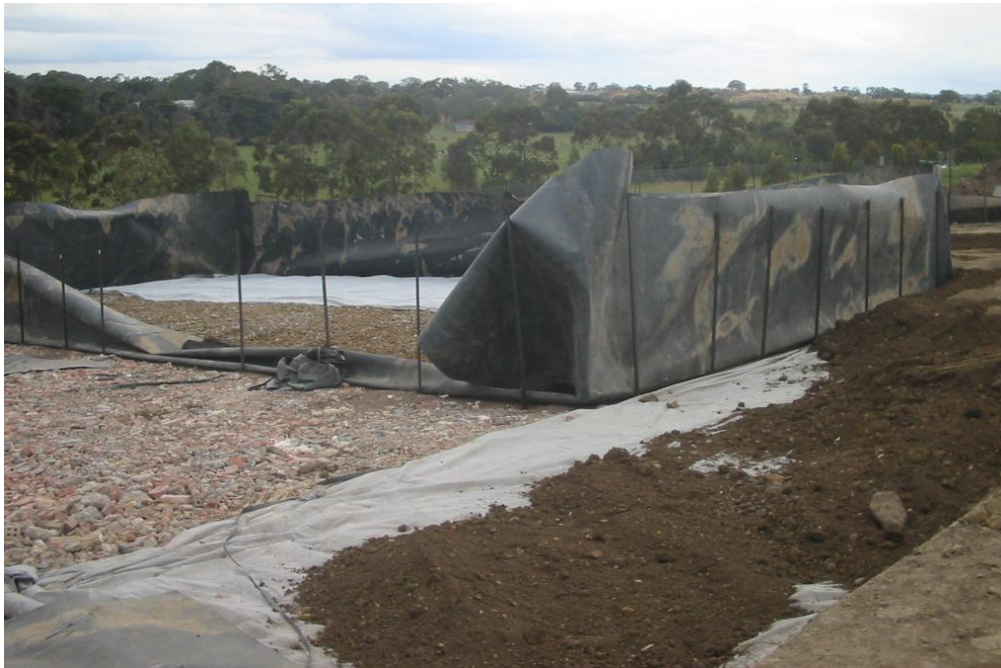
Figure 4.16 Phytocap Lysimeter Pan Supported by Star Pickets with Rubble Base and Partly Covered by Bidim™. First Lift of Sand:Compost Placed Outside Lysimeter
