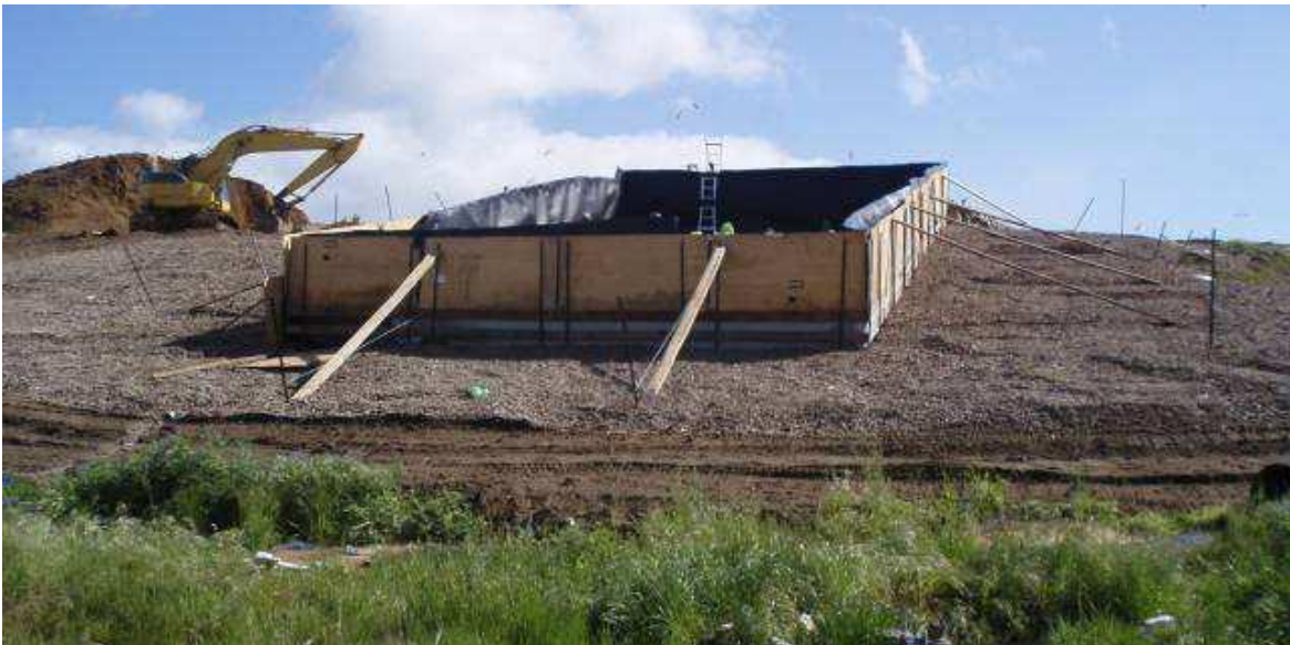
Figure 4.32 Lysimeter Box Erected on 25% Slope at Henderson Waste Recovery Park (Photo courtesy of IW Project (2010))
