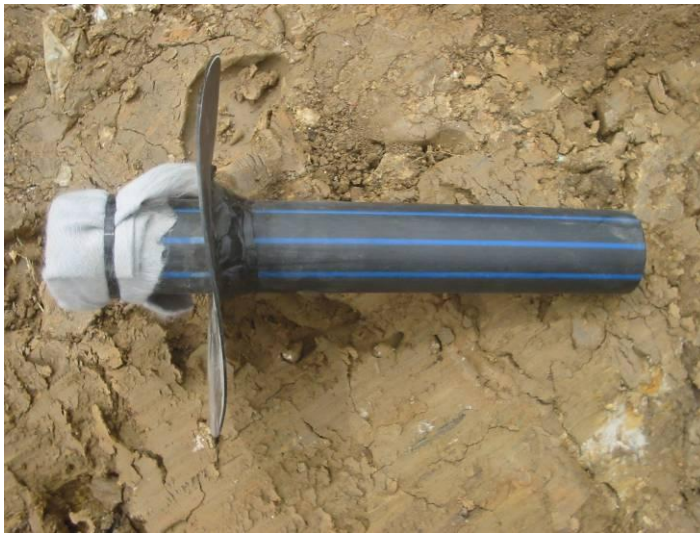
Figure 3.5 Welded Drainage Pipe (left) and Schematic Cross Section of Placement (right)
