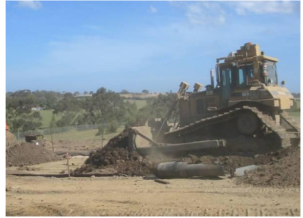
Figure 4.17 Construction of Conventional Lysimeter with Compaction using a Vibratory Padfoot Roller (left) and Placement by Dozer (right)
