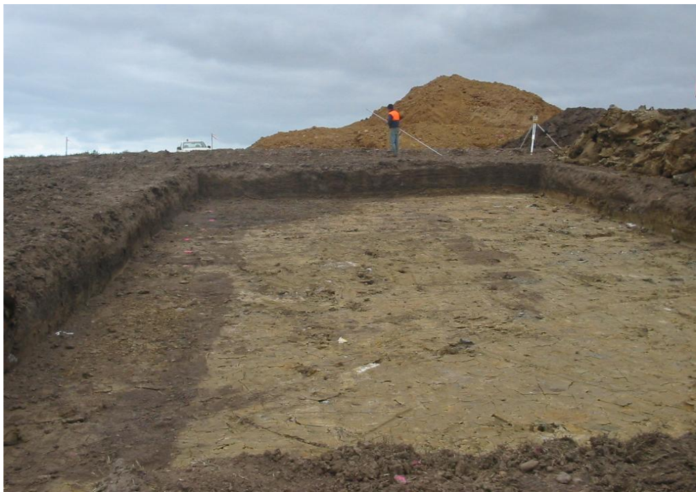
Figure 4.15 Excavation of Existing Conventional Cover for Conventional Lysimeter Construction.
