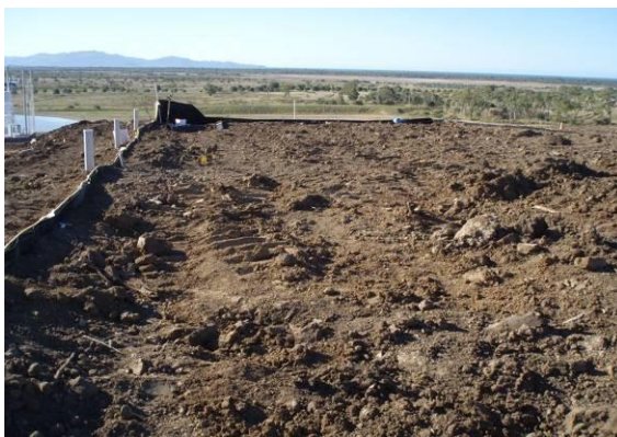
Figure 4.23 Phytocap Lysimeter (left) and Compacted Clay Barrier (right) During Construction (Photos courtesy of G. Zhu)
