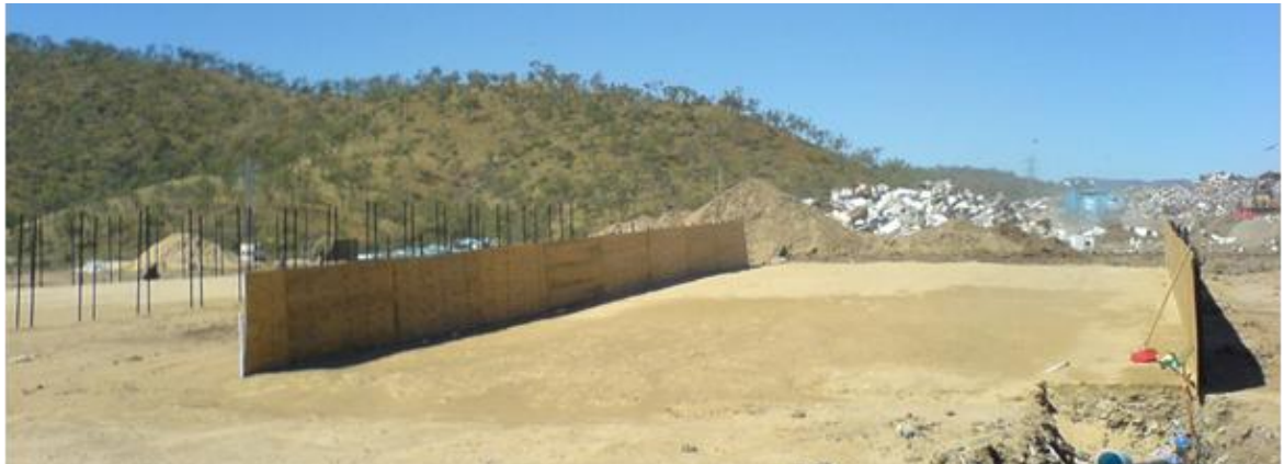
Figure 4.22 Sand Cushion Layer and Lysimeter Wall Support at Vantassel Street Landfill (Photos courtesy of G. Zhu)
