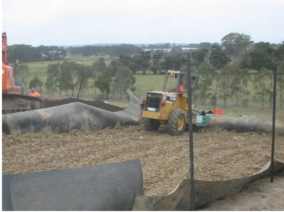
Figure 4.17 Construction of Conventional Lysimeter with Compaction using a Vibratory Padfoot Roller (left) and Placement by Dozer (right)
