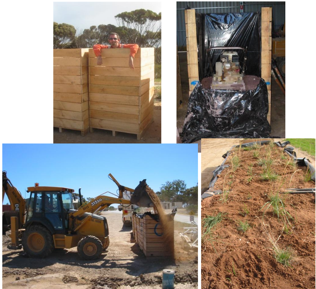
Figure 7.2 Construction of Small Plot Trial Boxes (top left) with Clay Compacted using a Vibratory Pad (top right) then Subsoil and Topsoil Tipped into Boxes (bottom left) followed by Planting (bottom right)
