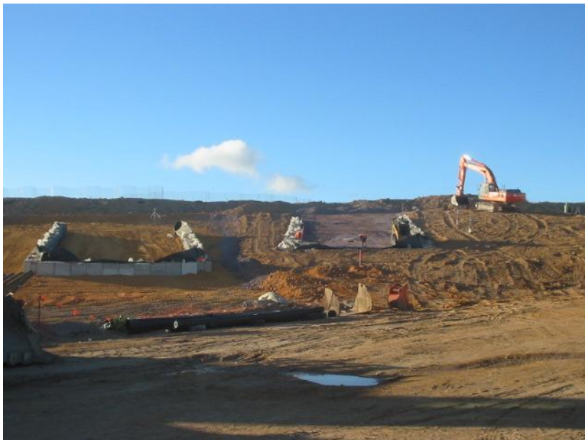
Figure 4.7 Silty Sand Base in Phytocap Lysimeter (left) and Purple Compacted Clay in Conventional Lysimeter (right)
