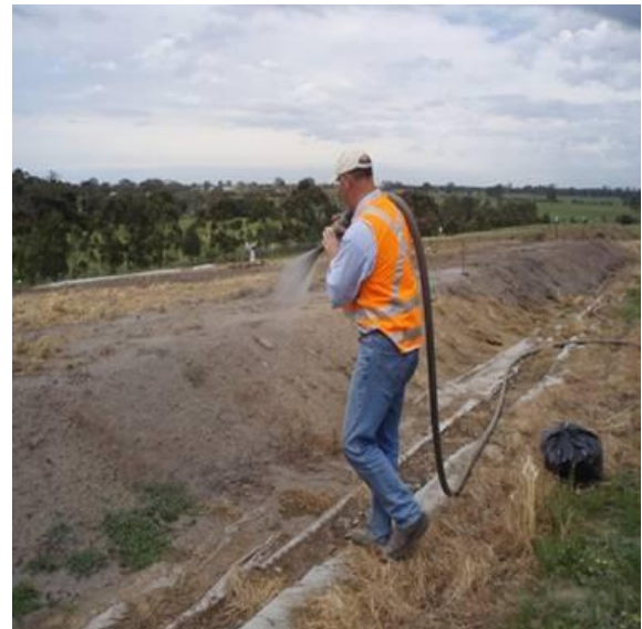
Figure 4.18 Planting of Trees and Shrubs in Phytocap Lysimeter (left) and Hydroseeding of Batters and Conventional Cover Areas (right).
