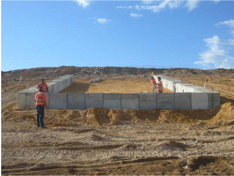
Figure 4.6 Concrete Blocks Used to Support Lysimeter Walls During Construction at SWD
