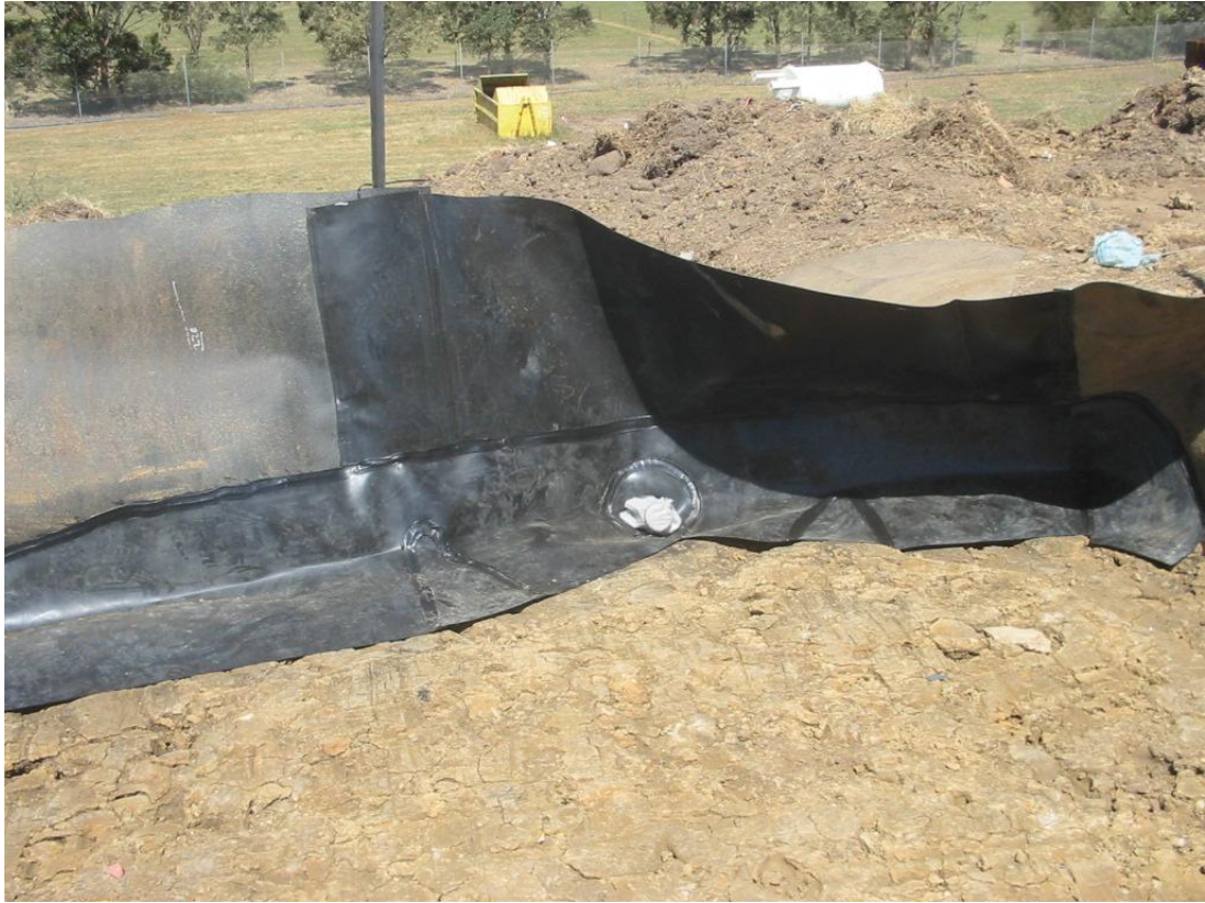
Figure 3.4 Lateral Flow Collection Flap and Collection Pipe
