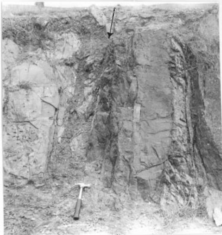
Fig. 53. Small E-W fault exposed in road cutting. Location C16. Looking west.
